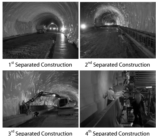
Fig. 1. Concrete Placement for Common Ducts by Human
